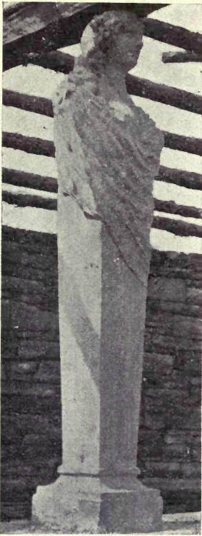
FIG. 97—ONE OF A NUMBER OF SYMBOLIC FIGURES IN CONCRETE, FORMING SUPPORTS FOR RUSTIC PERGOLA, ESTATE OF ALBA B. JOHNSON, ROSEMONT, PA.—ADOLPH SCHILLING
